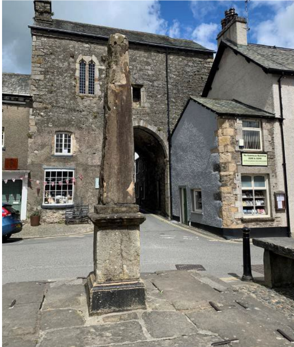
Figure 30: Historic surfacing in Cartmel includes sandstone flags and cobbles, which should be retained.
